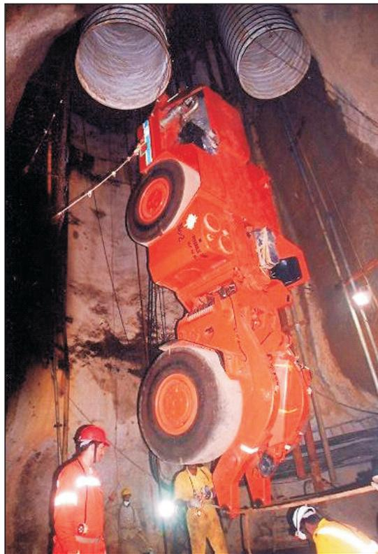
**FIG. 10 DISMANTLED EQUIPMENT BEING LOWERED THROUGH SHAFT**
