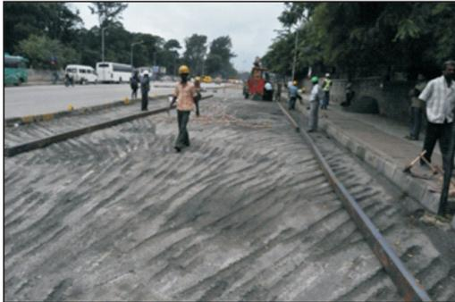
Surface preparation and alignment of rails for paver
